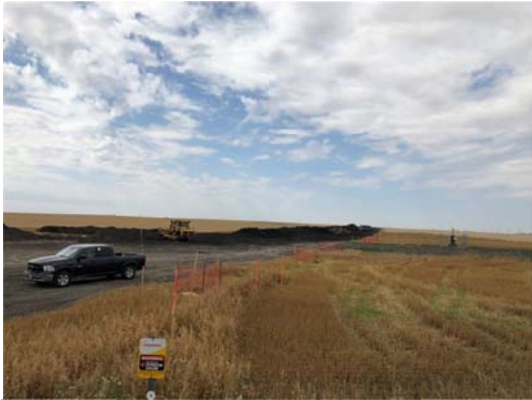
SF 42, west side, photo facing west, 6 dozers pushing dirt.
