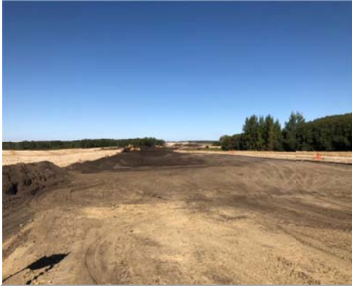
SF 38, half way through the ROW, photo facing west, top soil stripping.
