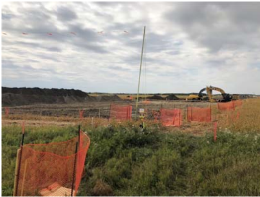
SF 41A, photo facing south west, excavators digging and some topsoil stripped.
