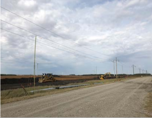
SF 48, photo facing north west, excavator moving dirt, crew preparing culvert in ditch, pump station is just on the other side of the road.
