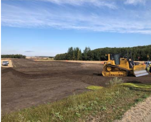
SF 38, (half way through) photo facing north west, dozer smoothing out approach.
