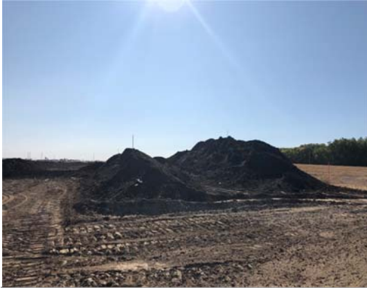
SF 38, half way through the ROW, photo facing east, dirt piles have been marked with stakes on the top.
