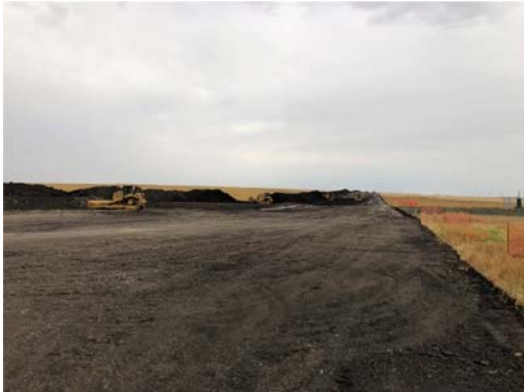
SF 42, photo facing east, dozers pushing dirt.
