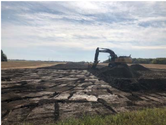
SF 38, (half way through) photo facing east, excavator pulling dirt to the side smoothing out the ROW.
