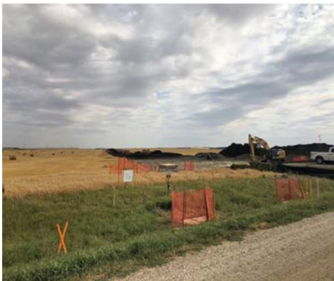
SF 41A, photo facing east, top soil being stripped by multiple dozers.
