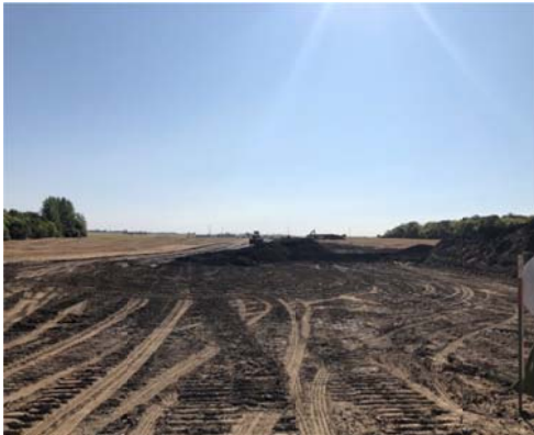
SF 38, half way through the ROW, photo facing east, top soil starting to be pushed to the side of the ROW.
