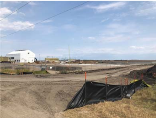
SF 48, photo facing north east, pump station.
