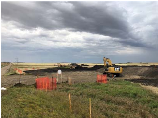
SF 43, photo facing south east, 2 excavators and 2 dozers pushing dirt.
