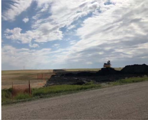
SF 43A, photo facing east, excavator piling topsoil.
