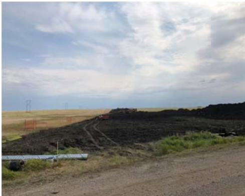
SF 43A, photo facing east, dozers pushing dirt all the way down the ROW.
