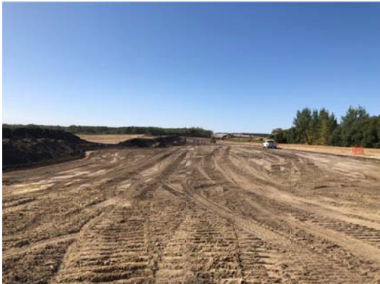
SF 38, half way through the ROW, photo facing west, top soil stripping almost complete, grader started grading.
