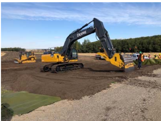
SF 38, (half way through) photo facing north west, excavator removing dirt from approach because topsoil was used instead of clay.
